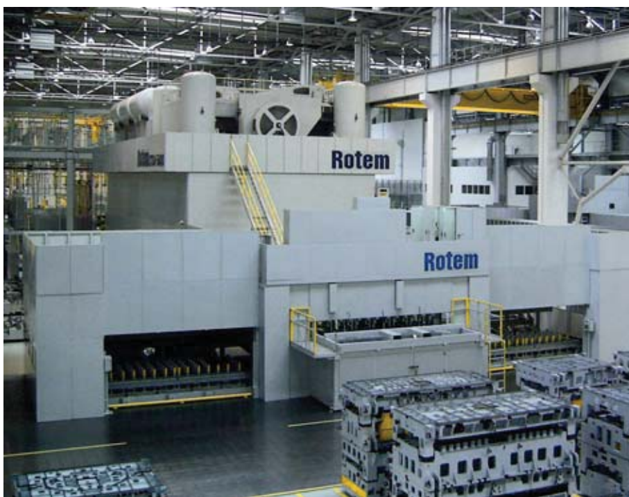
▲ Automation from a single source: KIA and Hyundai worldwide rely on components and solutions from Rexroth.
