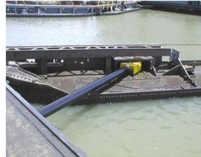
The hydraulic cylinder is attached to the miter gate. Bosch Rexroth's black Ceramax piston rod coating helps protect against corrosion.
