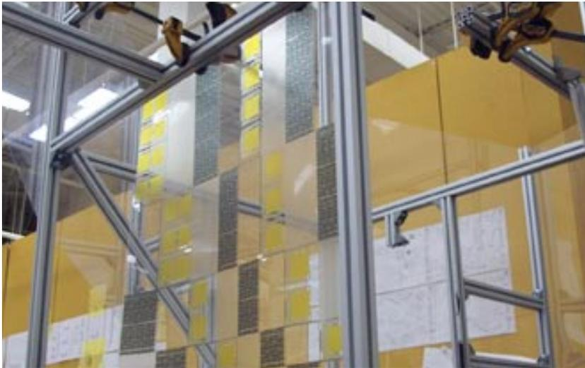
Aluminum structural framing offered the strength, ease-of-assembly, and aesthetic requirements for a complete, multi-functional SmartWrap exhibit structure.
