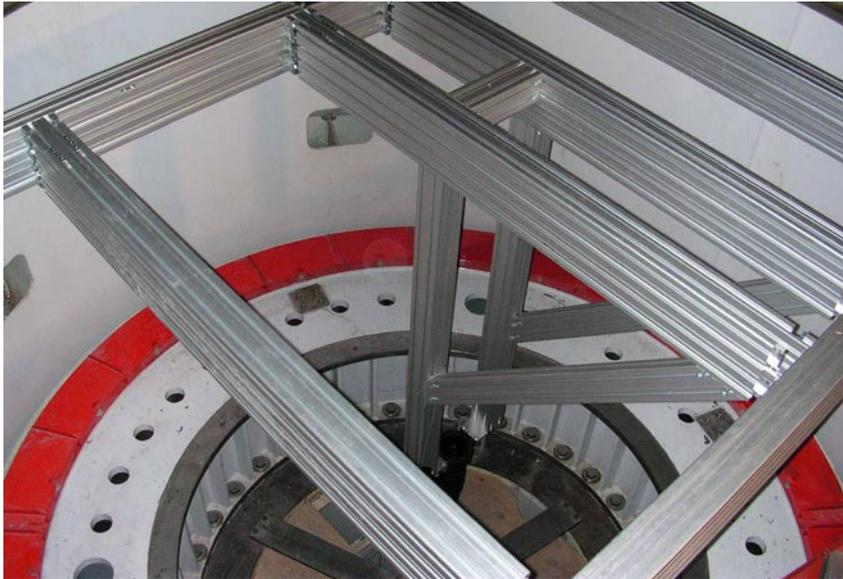
Project engineers used Rexroth aluminum structural framing to frame out the azimuth hole (above) before covering it with sectional steel plating and running the energy chain (below).
