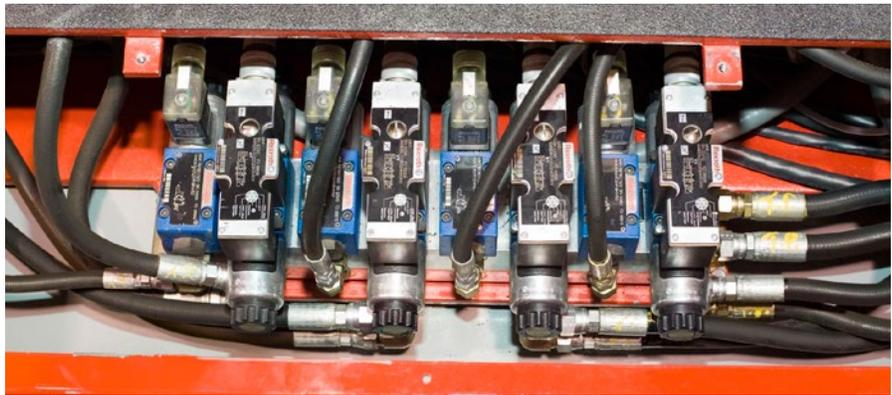
The K-RIG uses a hydraulic pump, and four Rexroth proportional directional valves and cylinders in each leg of the rig to lift the vehicle and provide the independent movement that simulates changes in the road surface.
