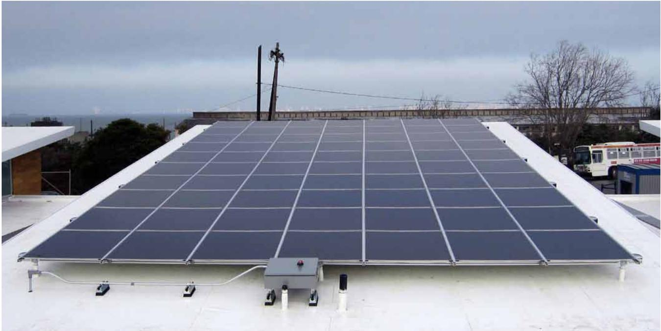
The mounting points were integrated in the Project Frog roof, which allowed the solar array to follow the roofline and slope to the south, improving the power output of the system.
