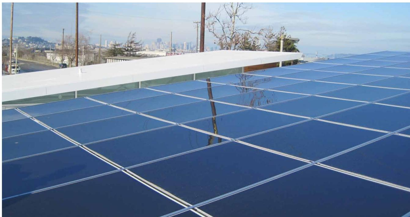
Working with Rexroth’s engineering team, Project Frog increased the length of the racking profiles to span a larger distance and bear directly on the trusses, which allowed them to drastically reduce the number of roof penetrations to 21 locations.
