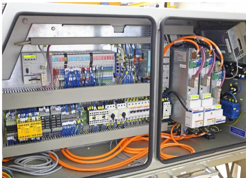
IndraDrive C compact drives enable high positioning accuracy and control.
