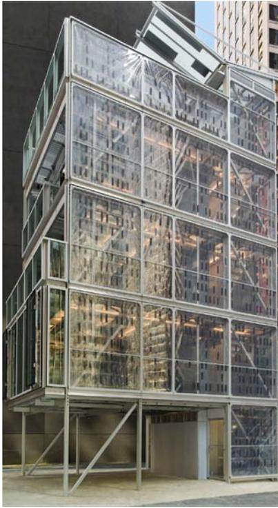
Cellophane House used lean manufacturing concepts and architectural ingenuity to create a new vision for mass customizable housing. The outer walls of the house consist of a thin film skin laminated with photovoltaic cells.
