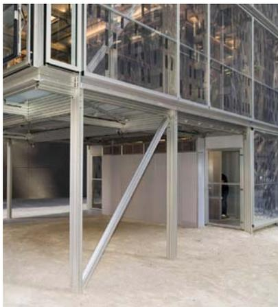
The frame of a multi-story structure experiences enormous forces in the form of shear stresses. KieranTimberlake’s hardware designs stood up to these forces which allowed them to change their entire approach to construction with Rexroth aluminum extrusions.
