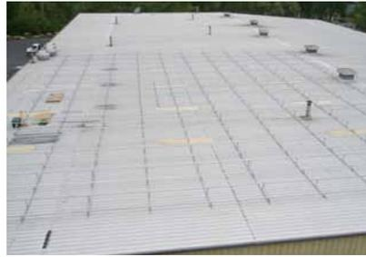
Straight aluminum profiles are now the basis of supporting solar panels in whatever configuration is needed, using simple tools and with no need for specialized training or even written instructions.
