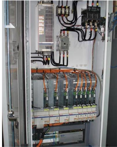
The Rexroth IndraDrive system and common DC bus with regenerative capabilities can divert excess power from one axis to another, or onto a mill's main power grid rather than dissipating that energy as heat.
