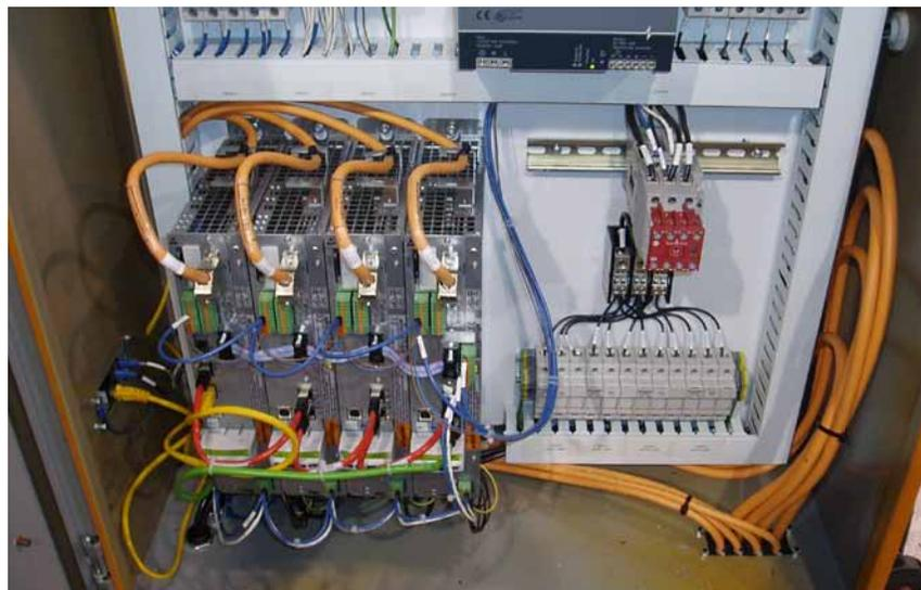
Specialty Tooling used a Rexroth IndraDrive MLD-M architecture with motion and logic combined in the drive to help reduce their wiring and control panel needs.
