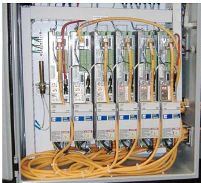
Ten servo axes are handled by Bosch Rexroth DKC servo drives which offer positioning block mode, angular and velocity synchronization, and cam functions.
