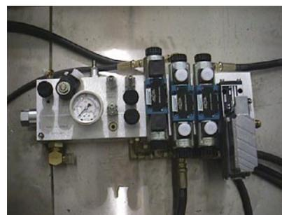
To solve the challenges of the previous D&S 5000™ design, the John Henry Foster team proposed a 7-1/2 HP electric motor powering a 6.5 GPM Rexroth gear pump and a two-station series D03 manifold.
