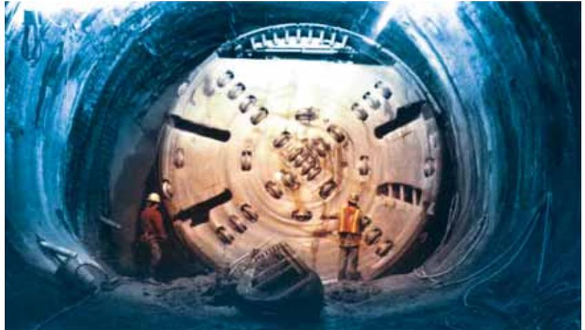
**New hydraulics from Rexroth helped CTS more than double the overall torque available on its tunnel boring machines.**
