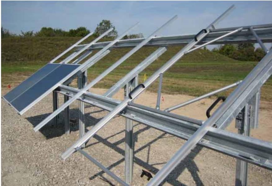
Rexroth's slide-in PV module mounting system securely encloses each module.
