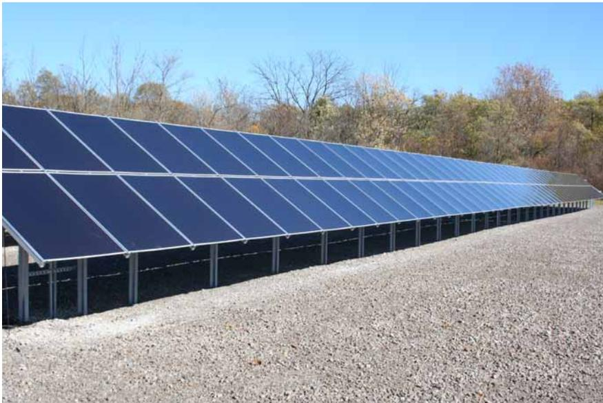
Bosch Rexroth's simple and effective slide-in mounting technology for micromorph thin-film solar module installation—including a base frame, plastic insert and rubber-coated stops—contains far fewer parts and cuts installation time in half compared to traditional installation systems.
