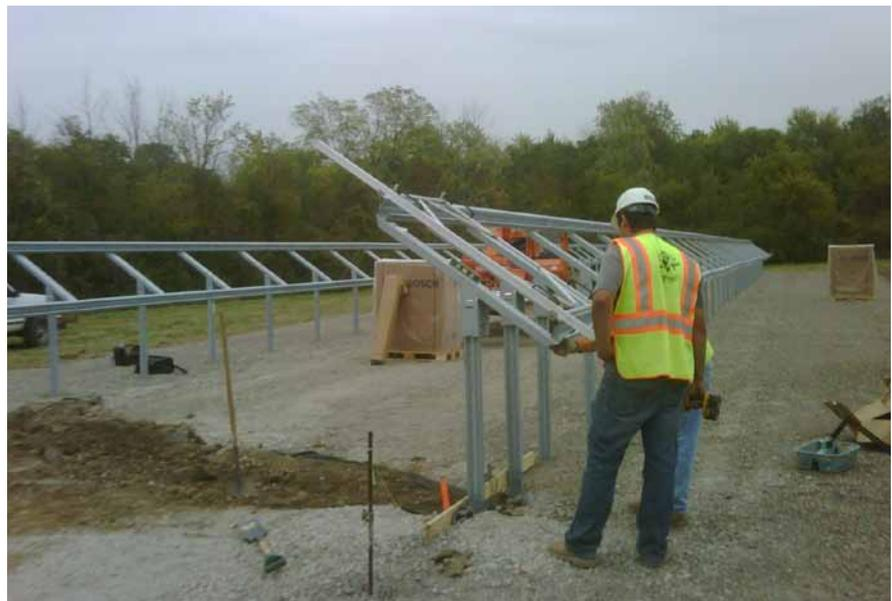
The framing system is easy to install. Once the initial framing is in place, the PV modules are simply slid into place. The end result is quicker installation with a durable frame that's rugged and weather-resistant.
